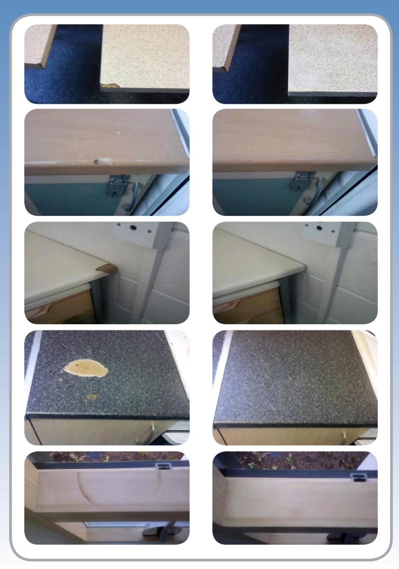
building back the surface using Ultrapremium filler. The area is then smoothed using a graduation of abrasives before the repair is colour matched, often with the Finisher mixing pigments by eye, and touching in details like wood-grain patterns using a fine artist's brush.
